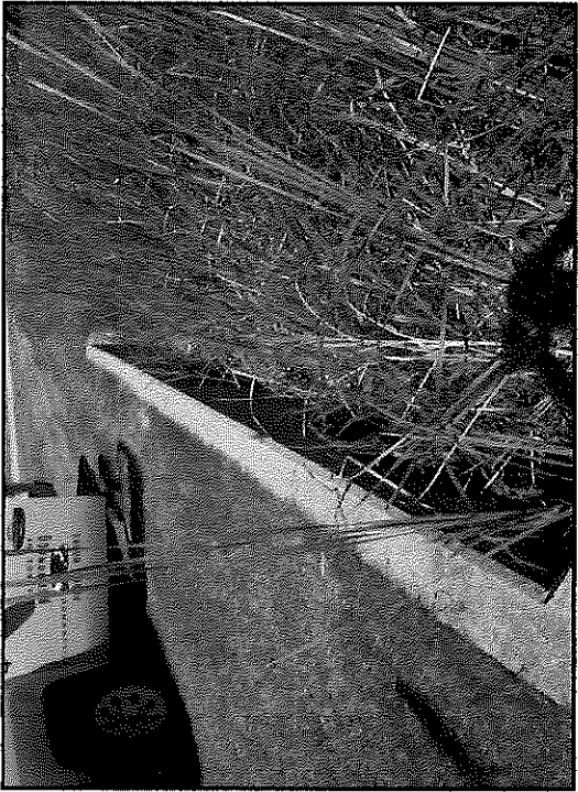
Outfall of culvert passing under Holz Pkwy...
