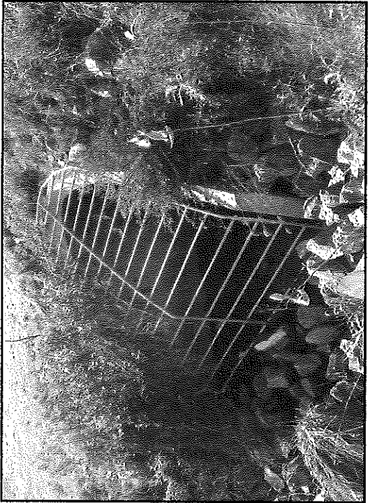
Outfall from Walmart, Home Depot pond
